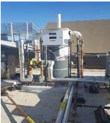
Examples of Outdoor OptiTherm Installations
